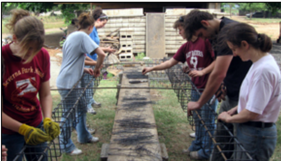
Bucknell brigade wiring rebar for posts
