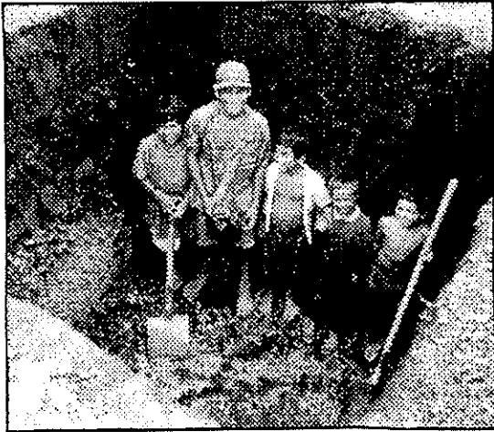
Children dig feeding center septic tank.
