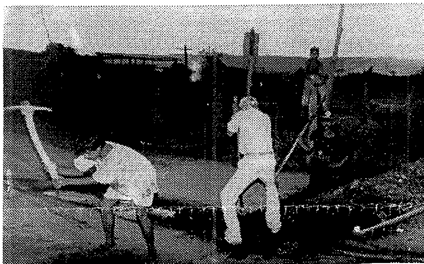
Using JHC donation to lay water pipe in Roberto Clemente
